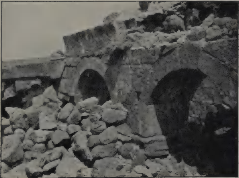
FIG. 318.—Tchauderlik, arcade between nave and N. aisle.
